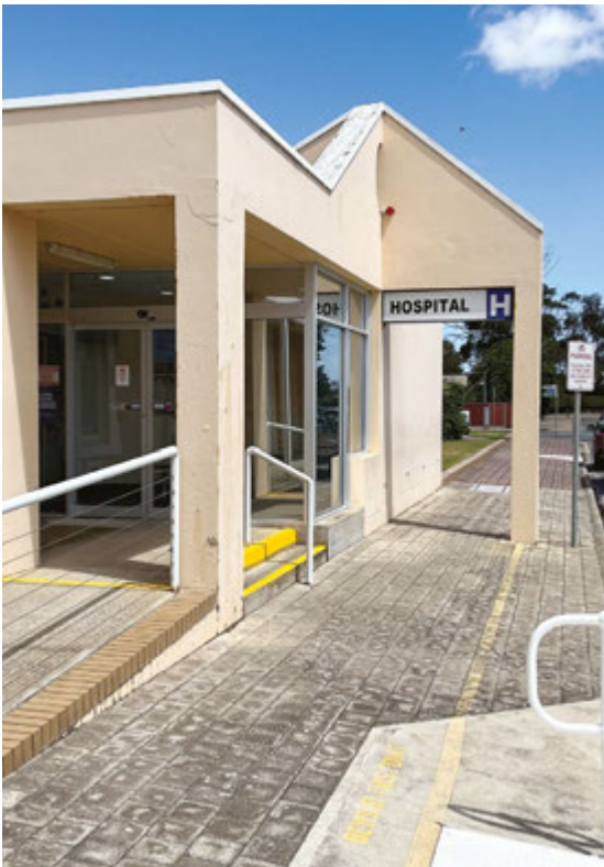
SERVICES NEEDED.... The Yorke Peninsula health services inquiry recommended that the development of an emergency department at Yorketown Hospital be investigated.
