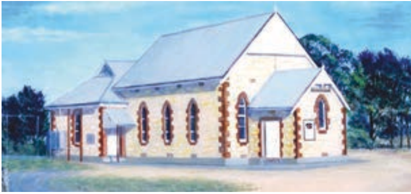
DEMOLISHED... Sandilands Uniting Church, as painted by Joy Davey in 2008; the dilapidated church and hall have had to be demolished due to safety concerns.
