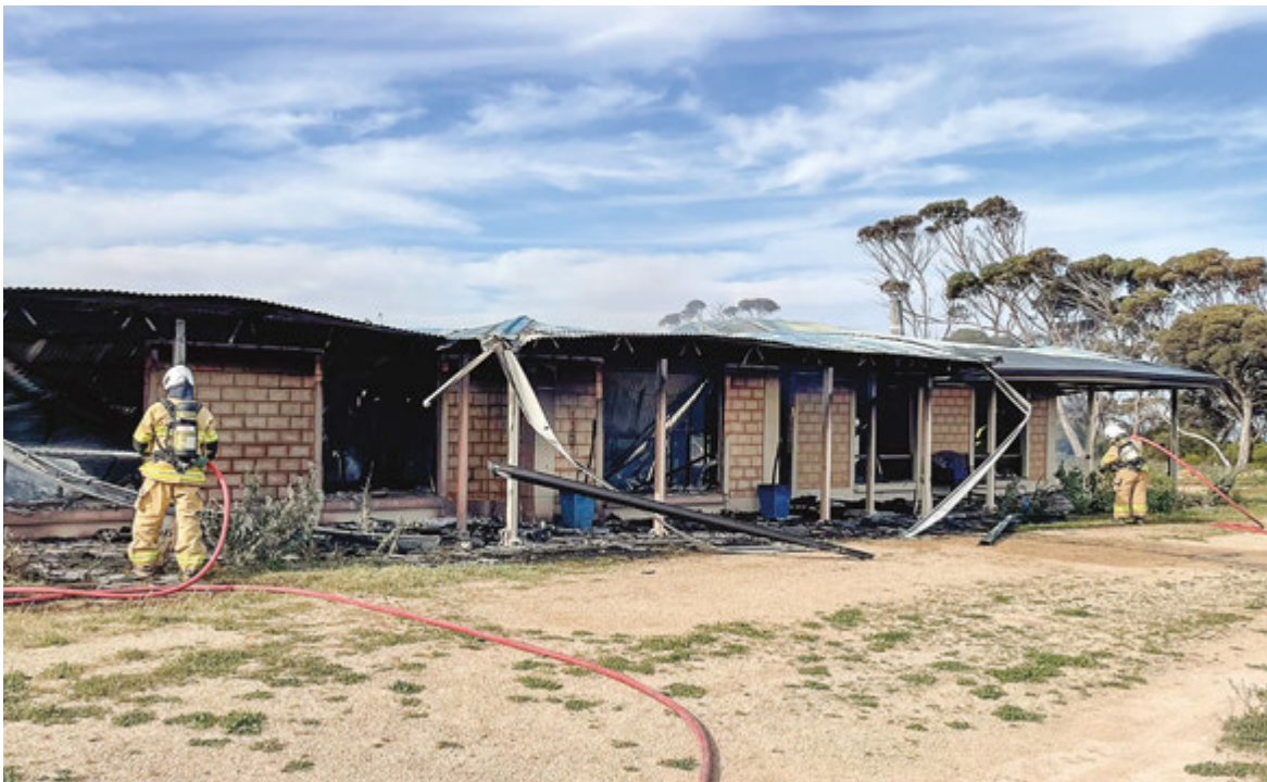
UP IN SMOKE... About 50 firefighters attended the blaze which destroyed this Clinton home.
