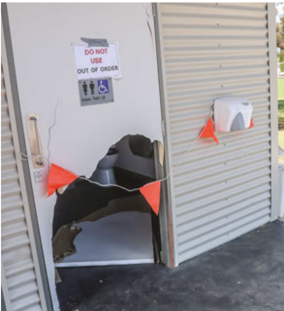
DAMAGE... A toilet door at Newtown Playground, Kadina, has been vandalised.
