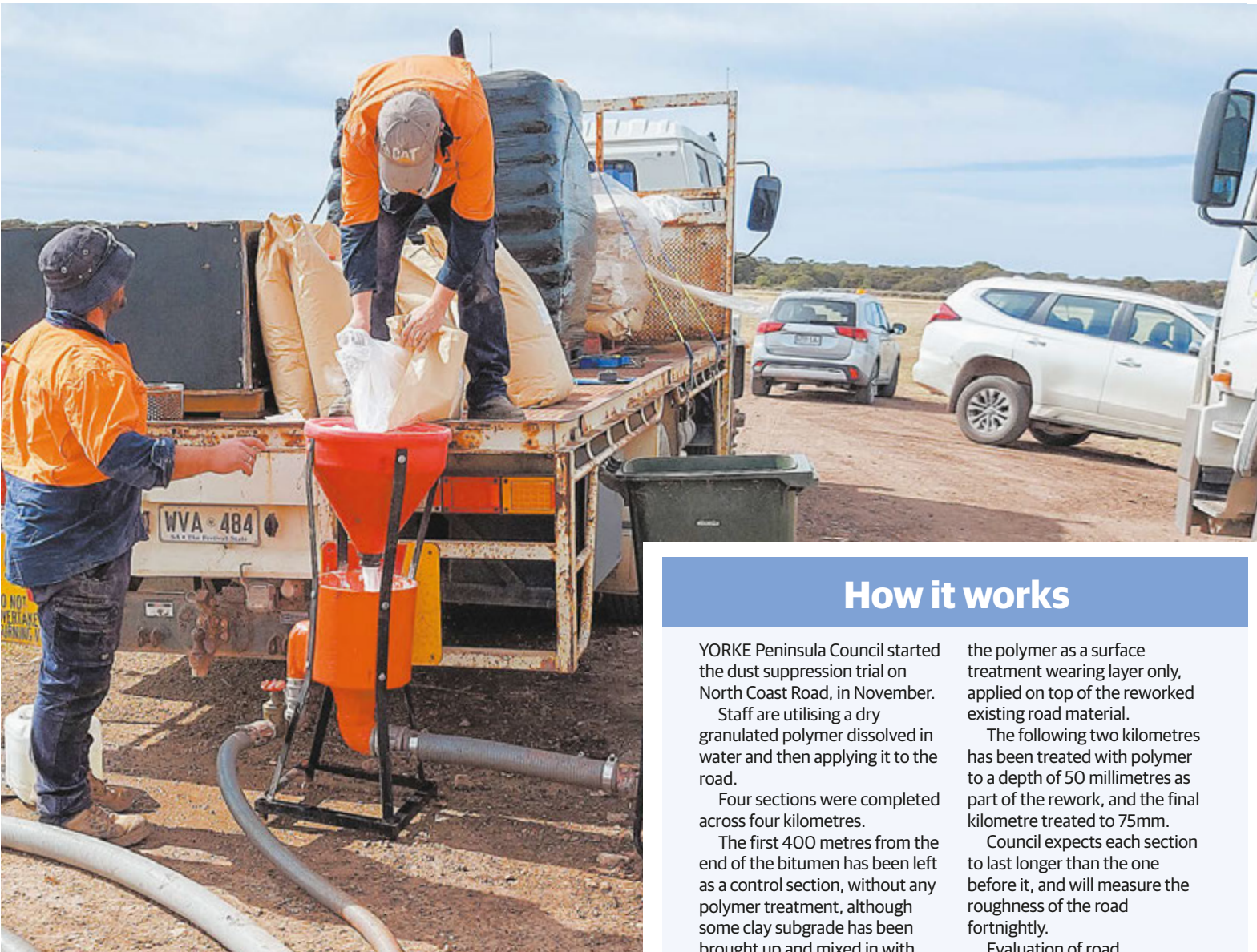
TRIAL... Yorke Peninsula Council staff Jayden Rice and Chris Baker mixing product ready for a dust suppression trial for North Coast Road in Point Turton.
