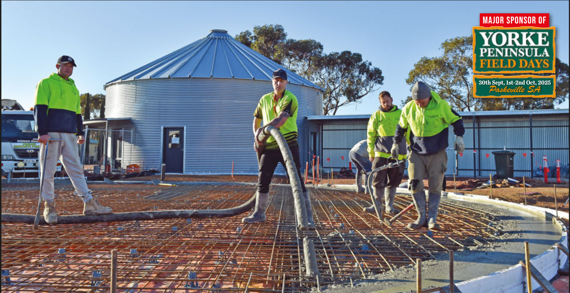
CONCRETE POUR... Local contractors lay the foundation for the new YP Field Days function centre.
