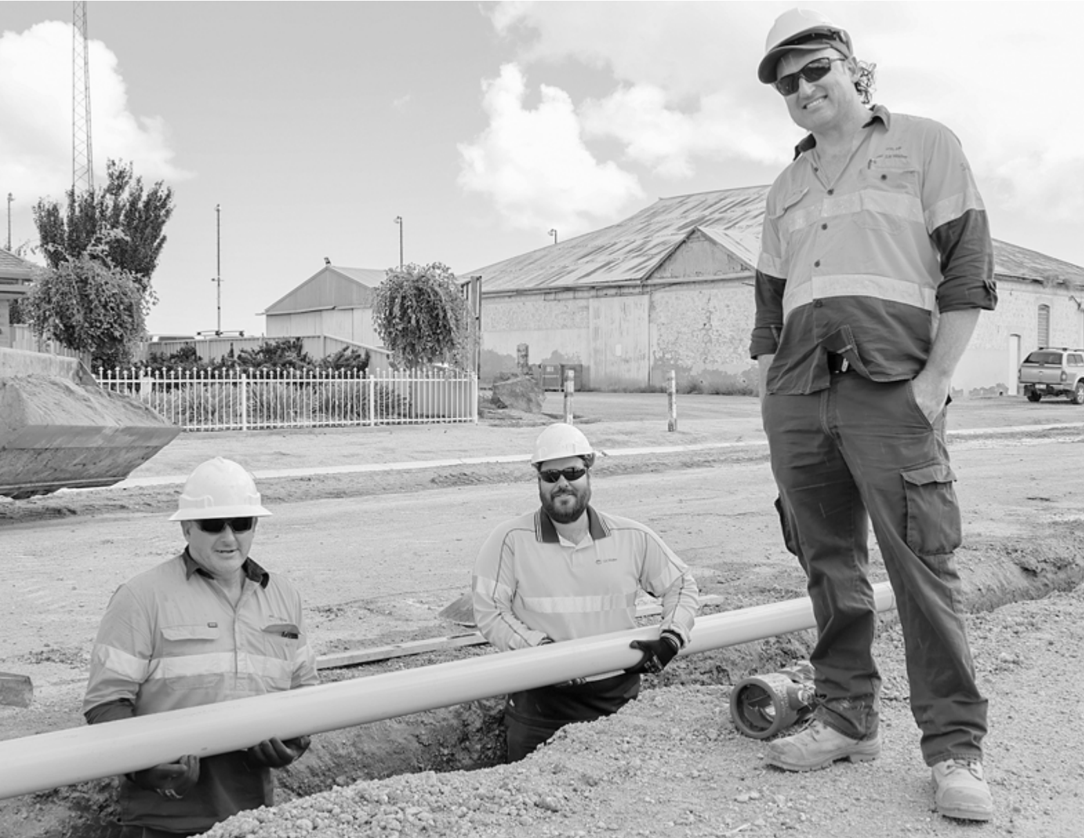
UPGRADE... SA Water contractors Bryan Kean, James Holloway and senior technical officer Dylan Champion lay a section of the 450-metre relayed water main along Agery Road, Kadina.
