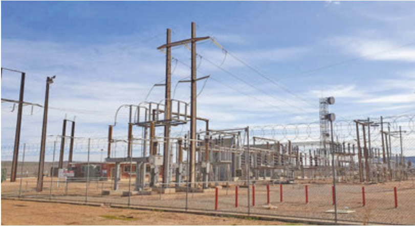
COMING CLEAN... The Hummocks substation was the source of an extensive blackout on March 14, caused by a build-up of salt and dirt on insulators during dry weather. ElectraNet held a planned outage for further cleaning on April 13.
