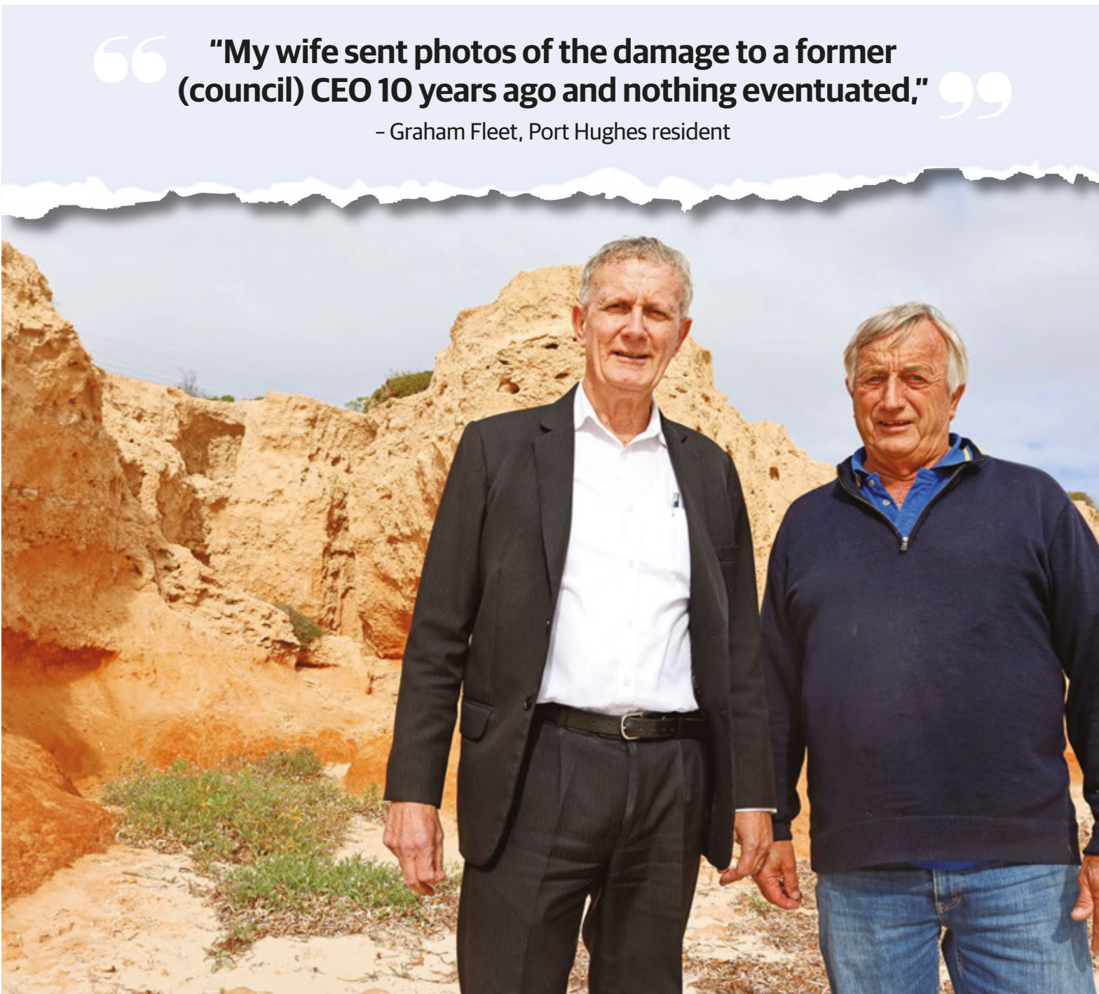
VITAL STEP... Copper Coast Council CEO Russell Peate and Port Hughes resident Graham Fleet hope $15,000 in state funding will help to identify a solution for an eroding Port Hughes cliff face.
